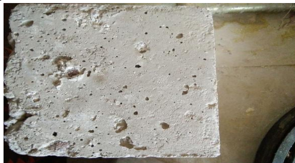
Figure 2: Alkali activated concrete cube after HCl exposure for 28 days (8 M)
