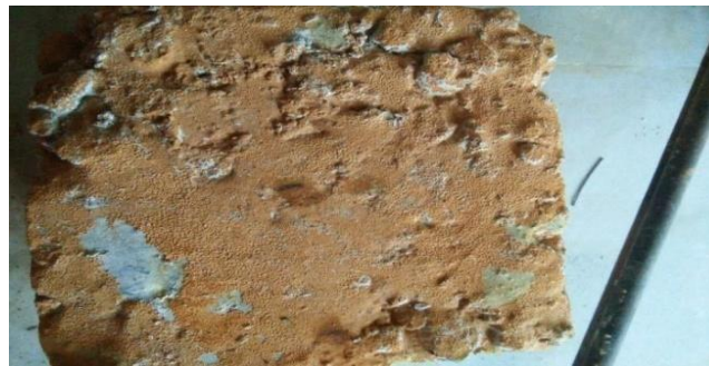
Figure 3: Alkali activated concrete cube after H 2 SO 4 exposure for 28 days (8M)
